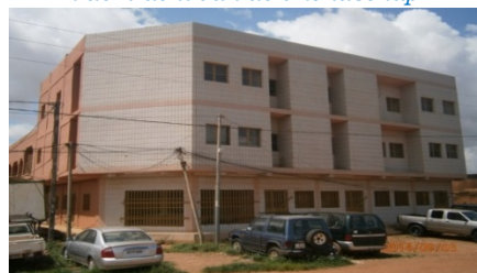
CPAEC in Ouagadougou Architect: Patrick de Louwere
